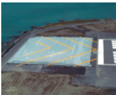
EMAS emergency arresting system at the end of the runway at Boston Logan airport (USA)
