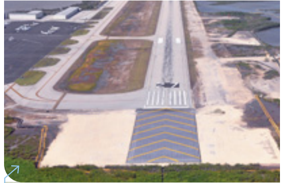
The EMAS system installed at Key West International Airport.
